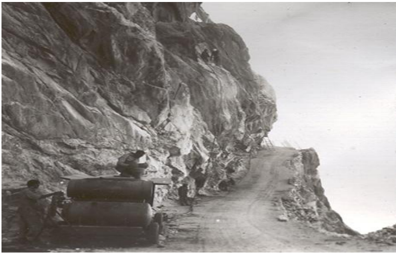
Figure No.6 Construction of KKH circa 1970
