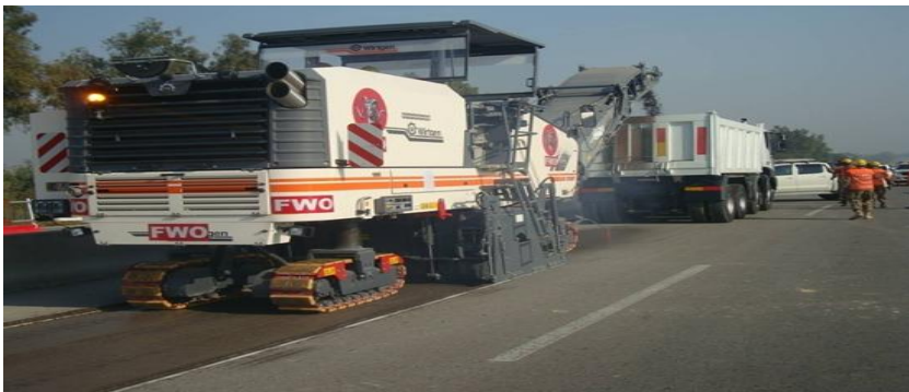
Figure No.15. Construction of Lahore-Islamabad Motorway (M-2)
