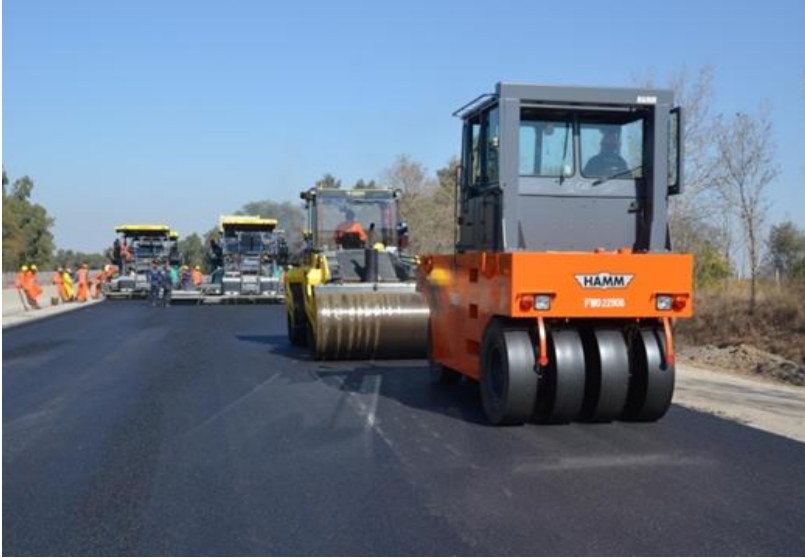
Figure No.16 Motorway Construction
