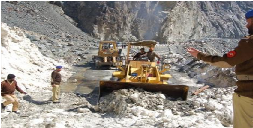
Figure No.7 Maintenance of Mountain Roads
